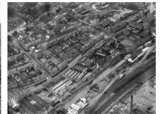
Huddersfield Street, Waverley Mill
